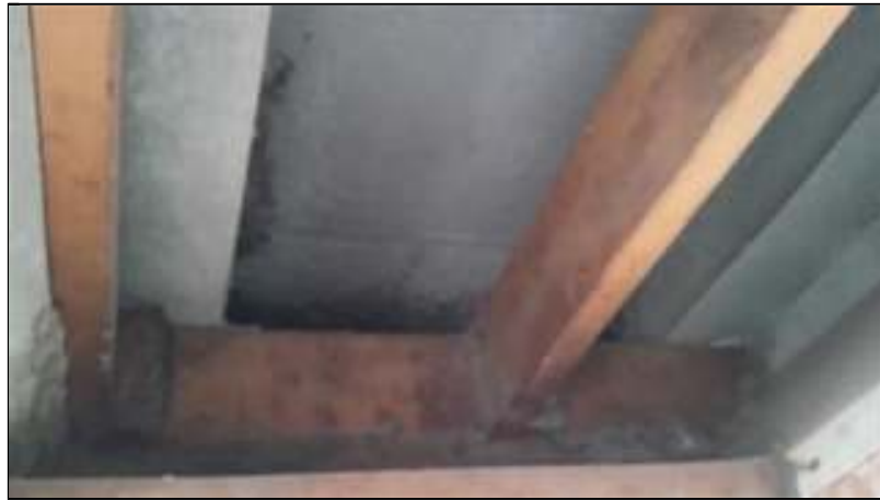
4.1 Item 2(Picture) thick dust in duct
